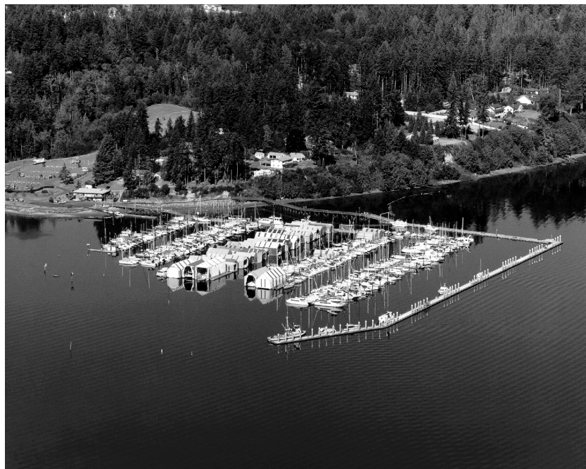
Figure 2. Photograph of the Marina With the Installed Floating Breakwater.
